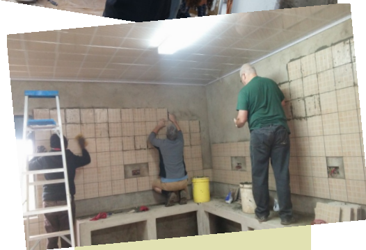
(ABOVE) PICTURES OF OUR TEAM DOING CONSTRUCTION AT THE HAVEN
