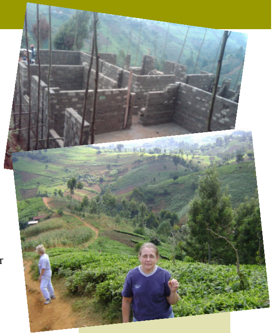
PICTURES OF THE HAVEN ON THE HILL CHILDREN'S HOME
